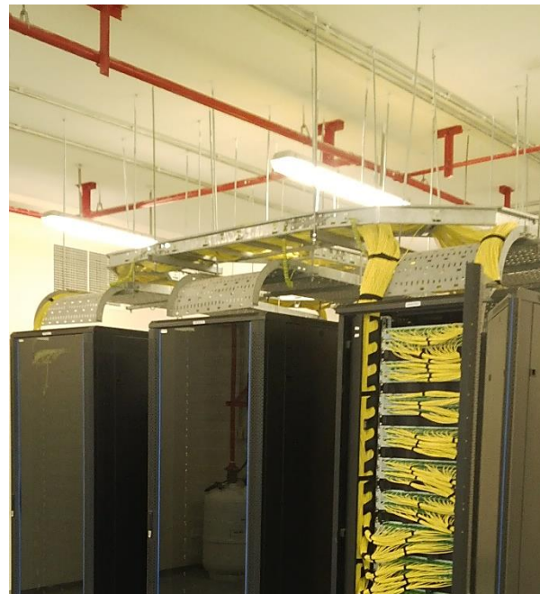
Photo 14.1d (Floor Telecommunication Room Cable Tray Layout example)
