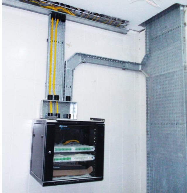
Photo 14.1d (Floor Telecommunication Room Cable Tray Layout example)
